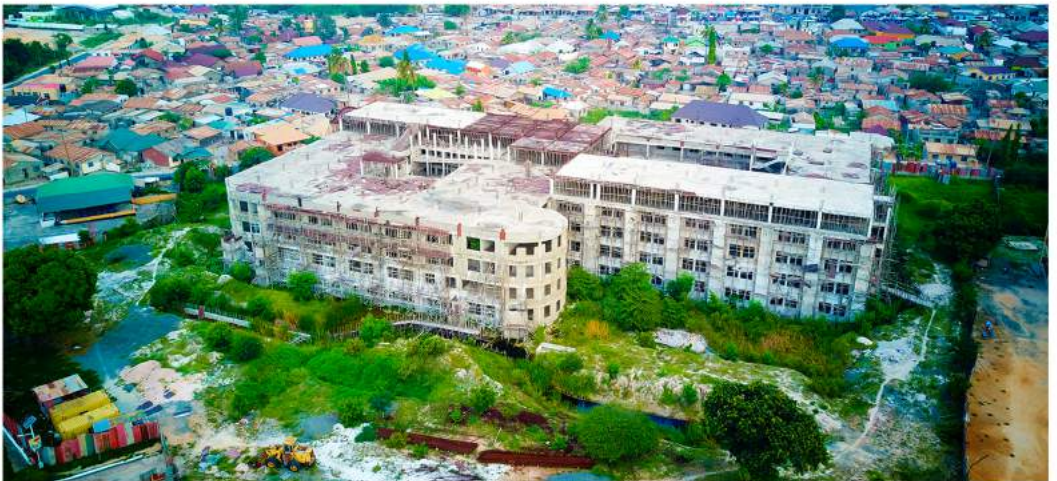
A view of the ongoing construction of the KIUT Teaching Hospital
